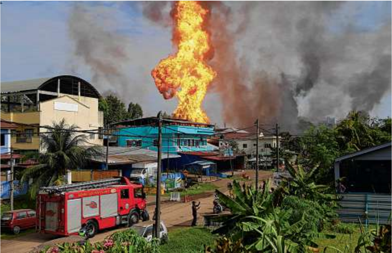
GAS LEAK: A massive pipeline fire forced evacuations in the Malaysian town of Puchong, outside Kuala Lumpur, on Tuesday.
