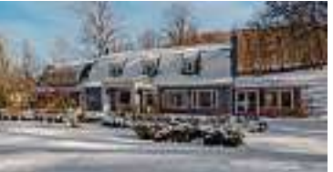
16 FOX HOLLOW LN. GARRISON, NY Country Carriage-style home offers charm and natural light. Stone walls, gardens and pool. $2,095,000 | M 845.661.5438
