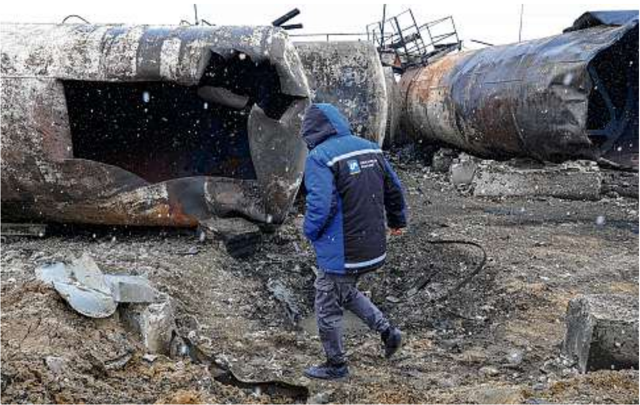
A worker inspected the damage at an oil refinery Tuesday, a day after a Russian drone attack, in Ukraine’s Kharkiv region.
