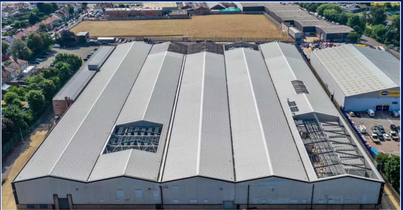
Green Mountain's 11,000m 2 Data Centre 'LON East'. Developed in partnership with TClarke. 30MW power capacity, delivering 1ms latency to the City
