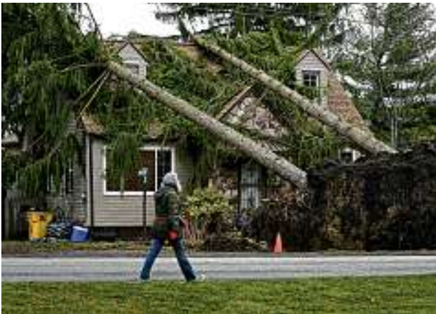
UPROOTED: Storm damage seen in Richland Township, Pa.
