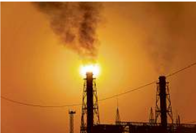
The U.S. waiver had allowed Iraq to address its electricity needs by buying power and the gas for generating it from Iran.
