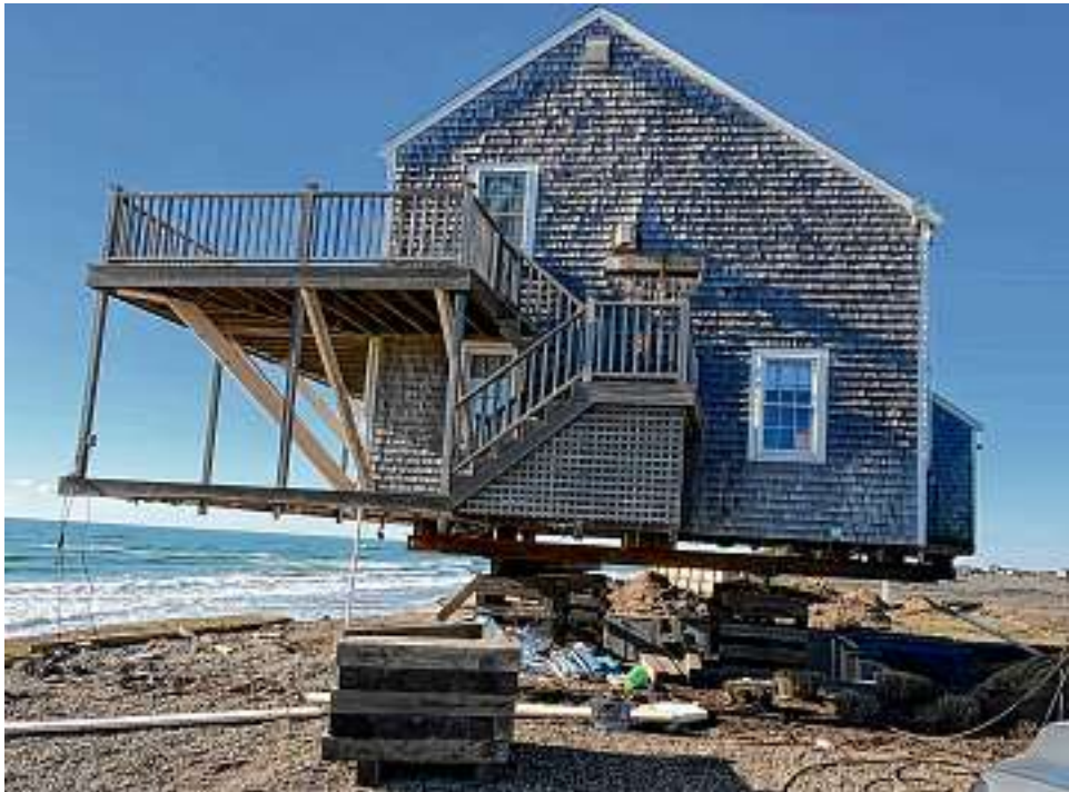
Above, a portion of Sheep Pond Road has been compromised by erosion. Left, a house was condemned a day before it was to be sold at auction in December. It was put on steel beams and rolled about 200 feet back from the water’s edge.
