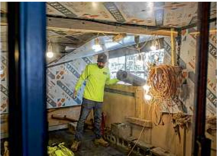
Left, wooden platforms along the house's south side will let workers repair the cantilevered 'shelf' above. Enclosures, above, are heated to keep workers comfortable and building materials at a constant temperature, at center.
