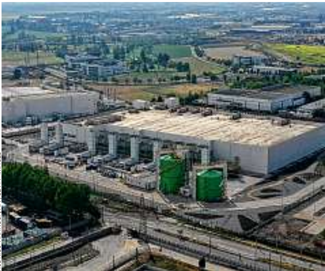
A data center in Santiago, Chile, that is owned by Google. Tech giants including Google operate 445 data centers in the U.S.
