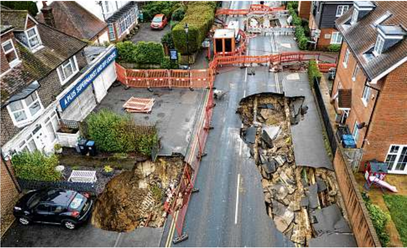
HOLEY TERROR: A pair of sinkholes appeared in Godstone, Surrey, England, after a water main burst, prompting evacuations.
