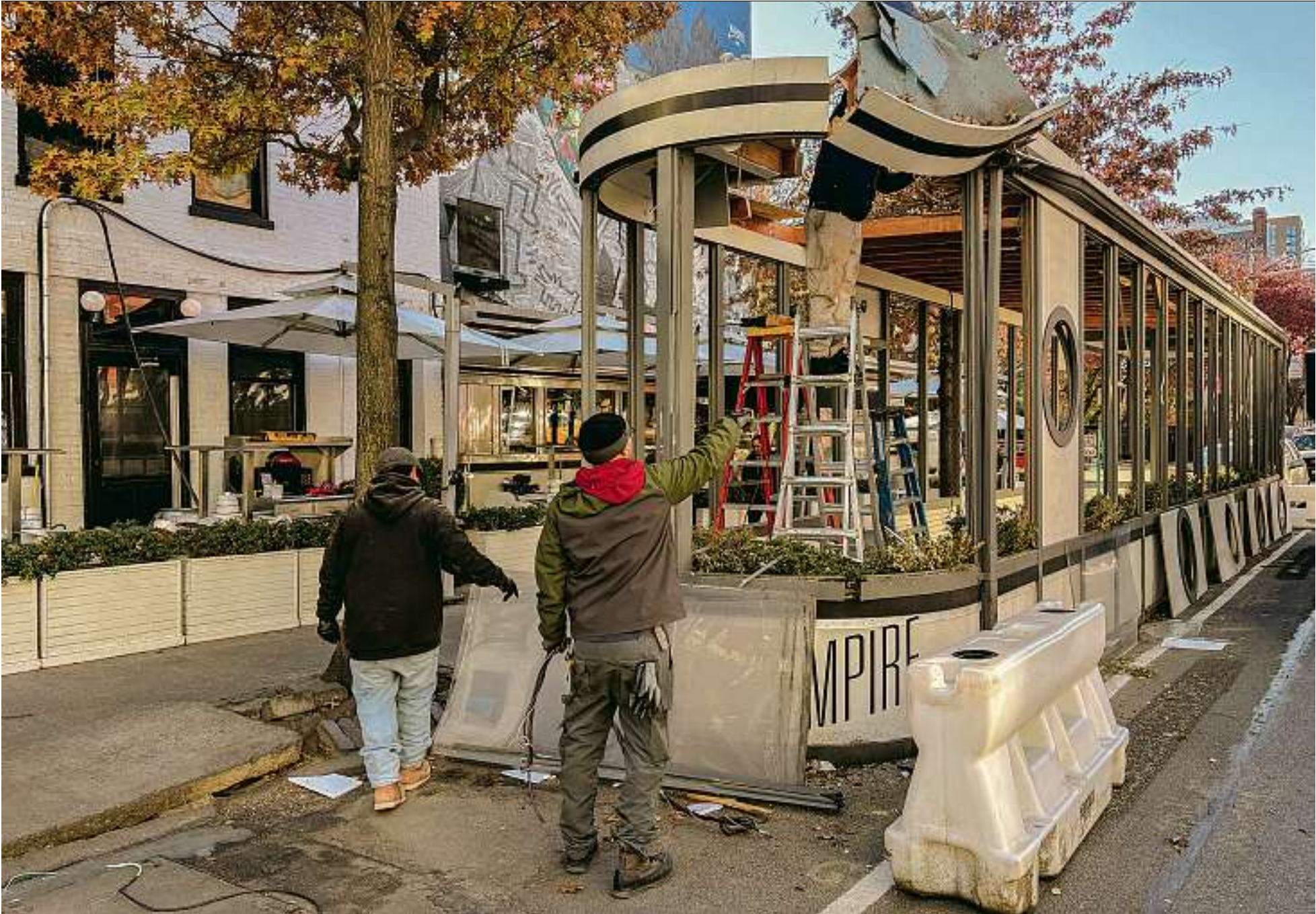
Workers dismantle the Empire Diner’s outdoor dining shed in Manhattan.
