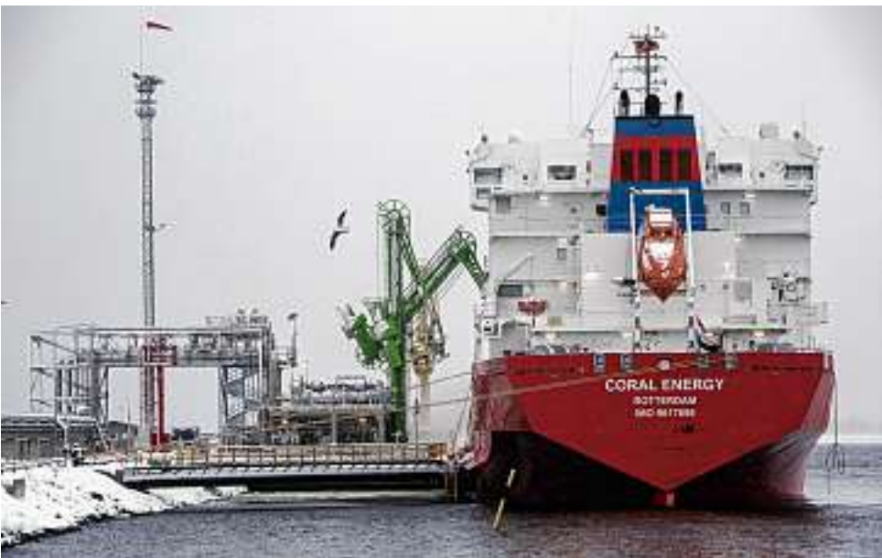
The first LNG ship arrived at the Manga LNG terminal in Tornio, Finland, in 2017.
