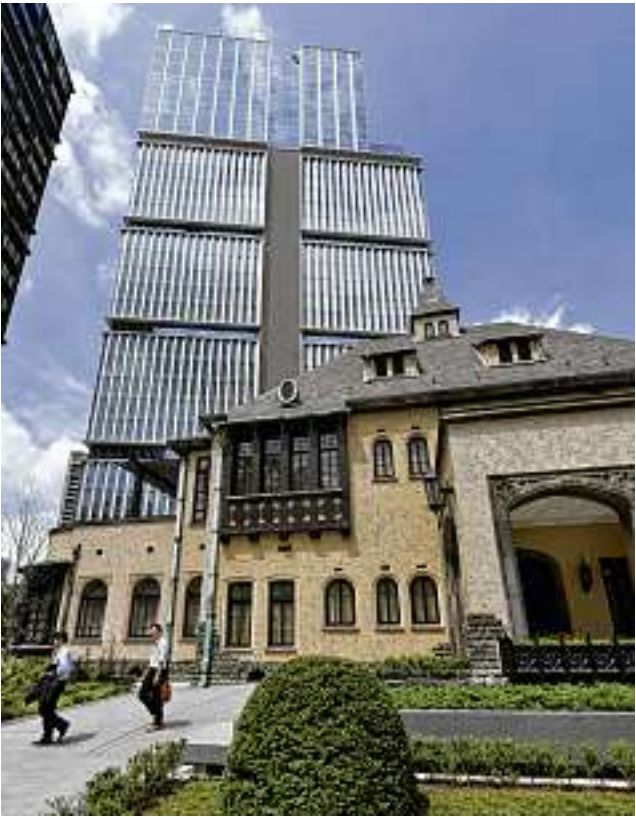
Tokyo Garden Terrace Kioicho includes homes and stores.
