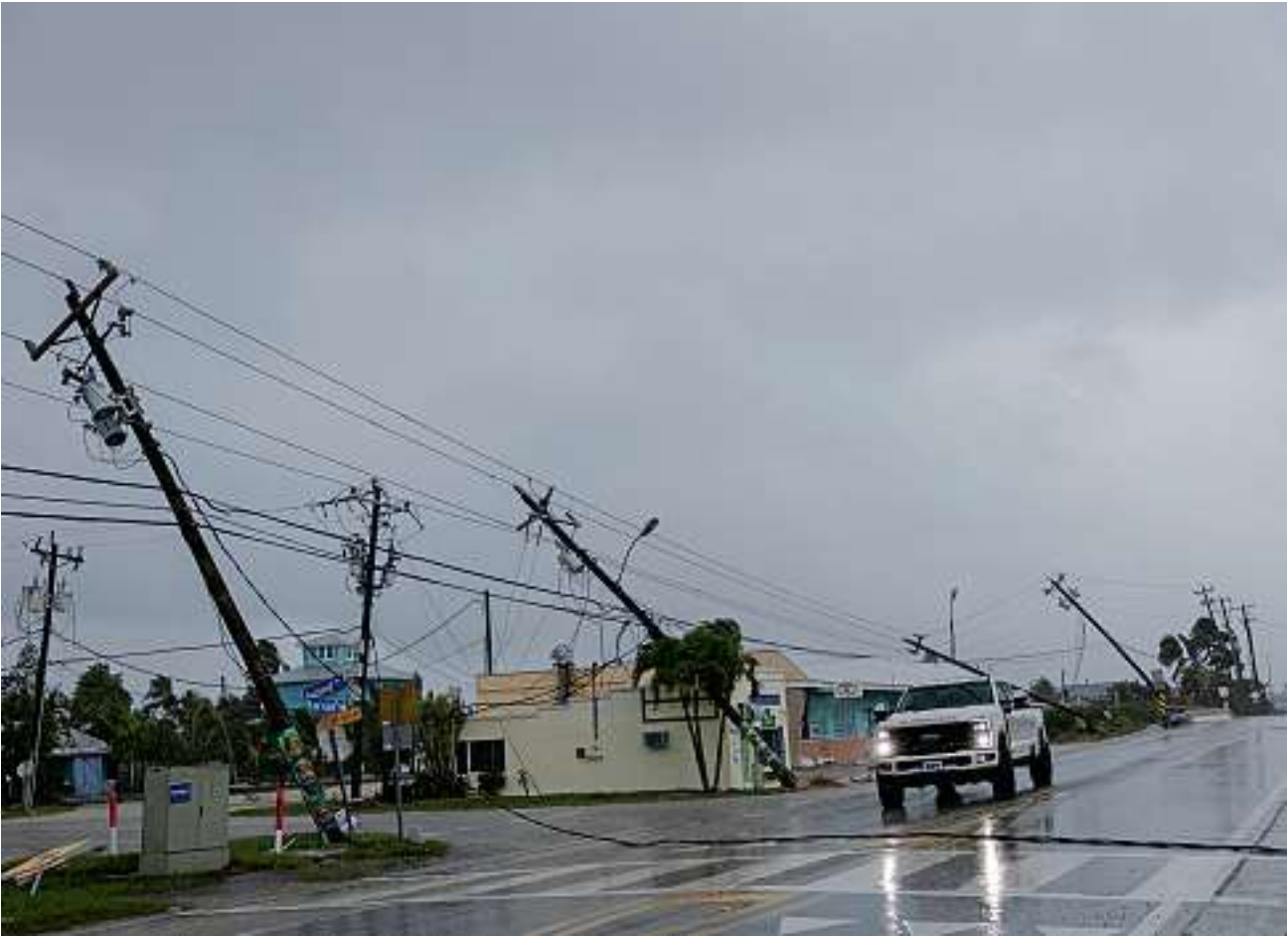
Utility poles were toppled by strong wind gusts in Fort Myers, Fla., before Hurricane Milton made its landfall Wednesday.
