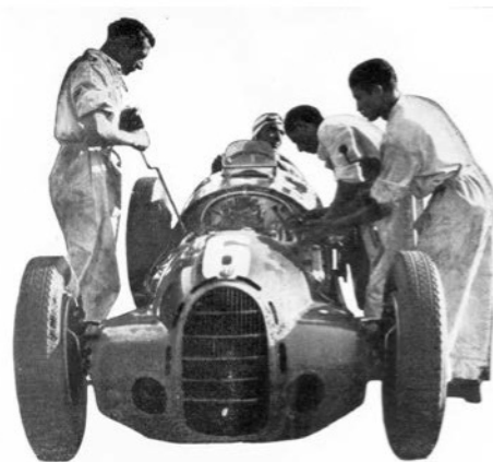
At an unidentified location, an Alfa 312 having its spark plugs changed. This model's front end had also received a number of alterations, seemingly aimed at improving cooling
