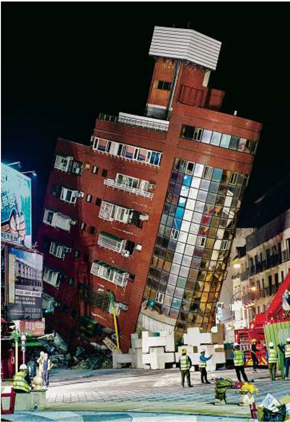
ROCKED: Emergency workers outside a partially collapsed building in Hualien on Wednesday, following a magnitude-7.4 quake that killed at least nine and injured 900. At least 130 people remained trapped, including 70 stuck in two mines operated by a cement company. A5
